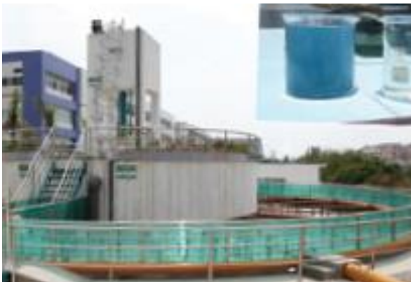
Figure 1: Yida Wastewater Treatment Plant (Crystal Group, 2011)
