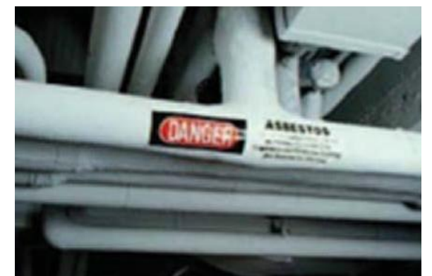
Good Practice: Asbestos-coated pipes are properly marked.
