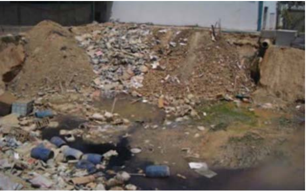
IA Bad Practice: Construction waste, garbage, chemicals, and discharge from pipe all commingling in one pond. All waste must now be treated as hazardous.
