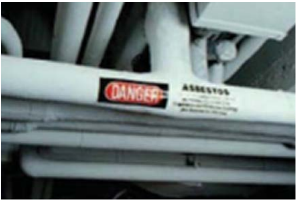
Good Practice: Asbestos-coated pipes are properly marked.
