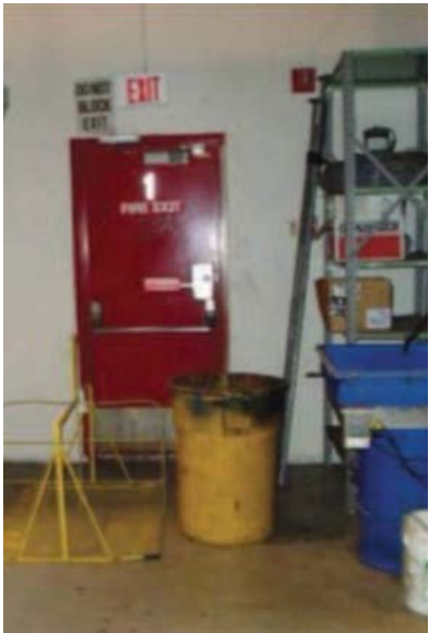
Bad Practice (IA): Fire exit is blocked by trash container and equipment
