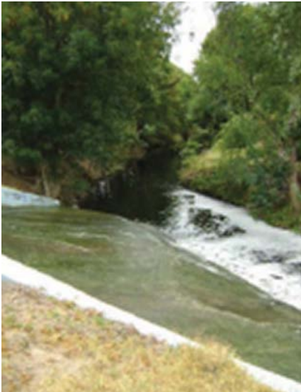
Good practice: Paving at point of discharge helps prevent stream bank erosion.
